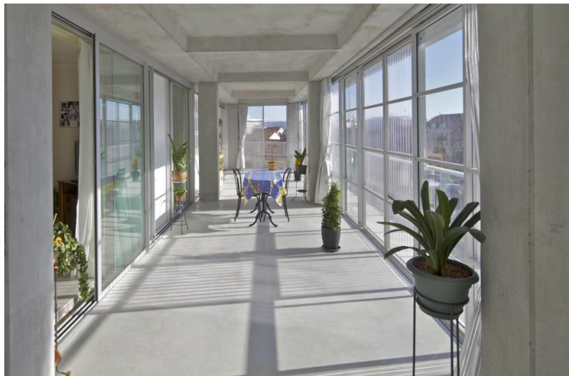
Figure 2. Renovation of the Grand Parc building in Bordeaux. Architects Lacaton & Vassal
